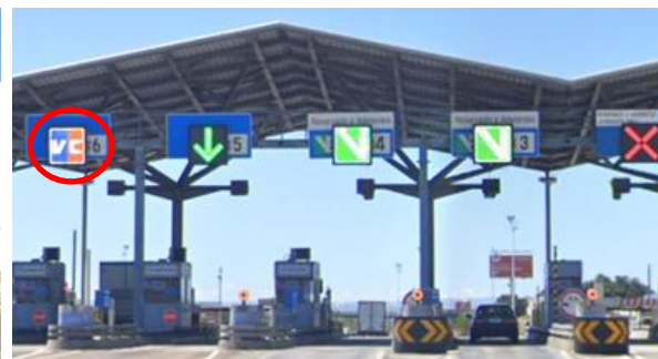
Ponte V. Gama (2025)
