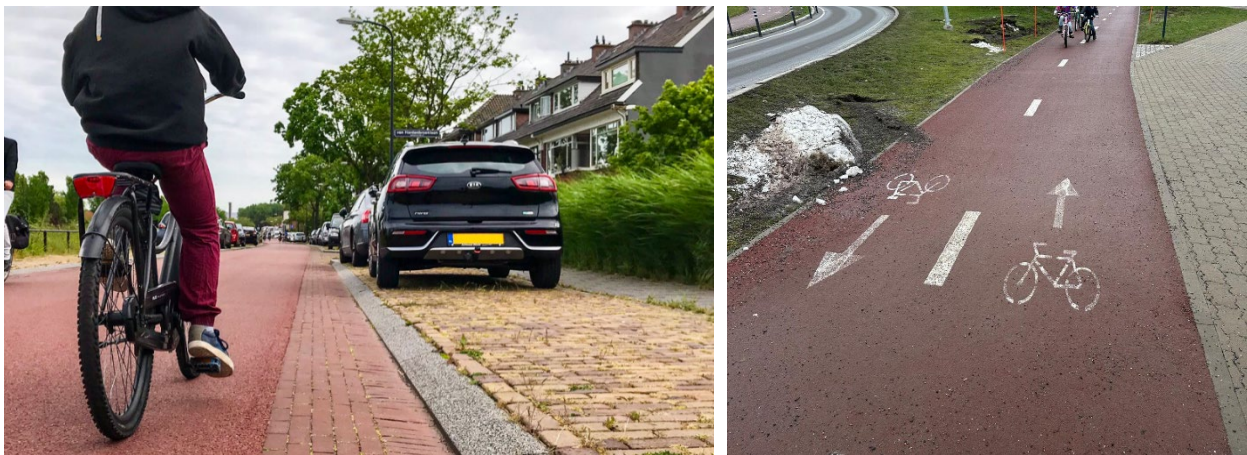
Fig. 8. Weeds in the brick openings [Dutch Cycling Embassy] (left), and wear and tear on the cycle path pavement ©Telko Estonia (right).
